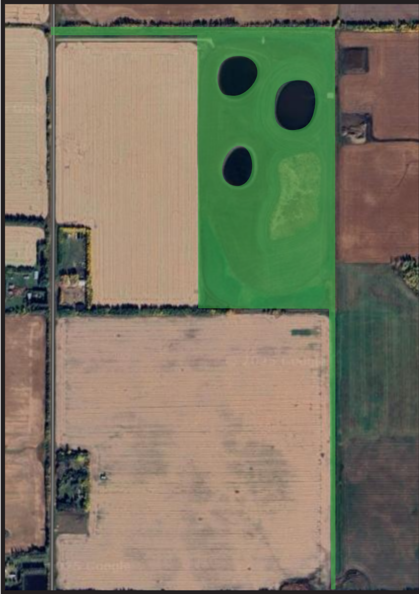
Three Lakes Stormwater Detention & Drainage Channels 28.7 ha
