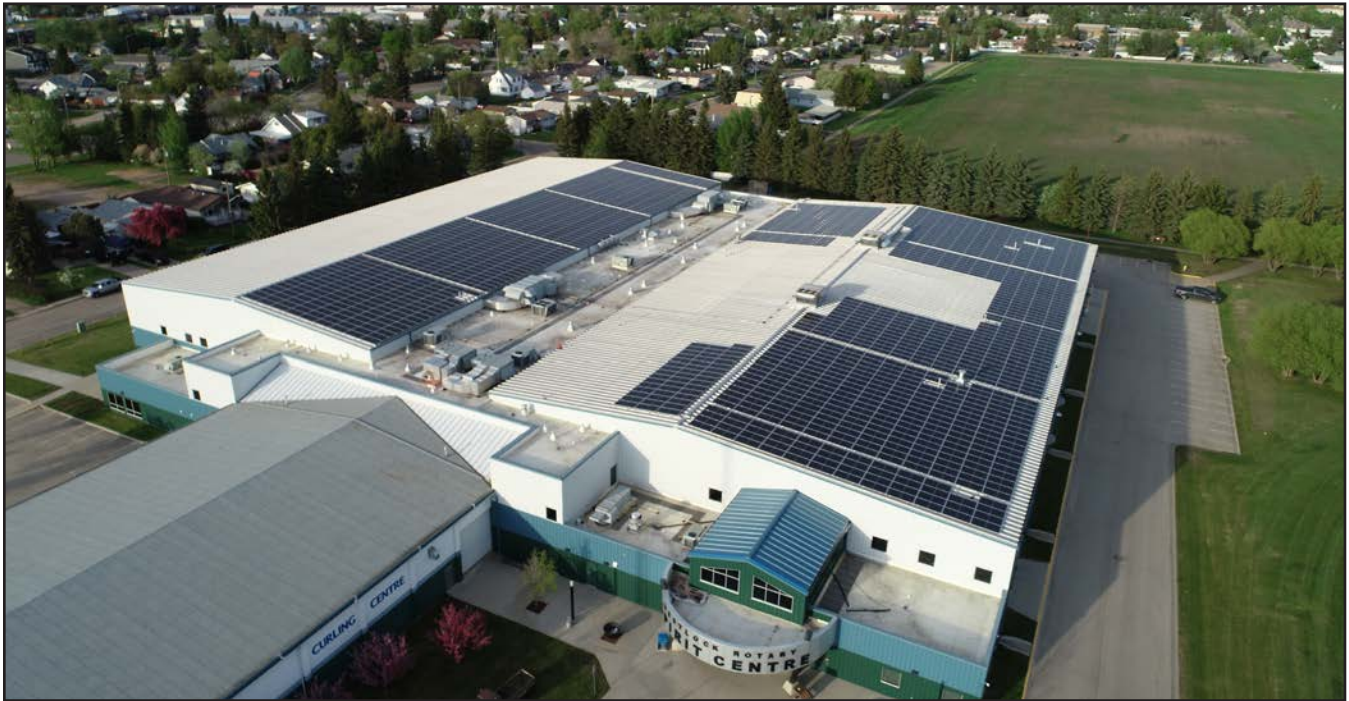
Westlock Rotary Spirit Centre, Solar Panels
