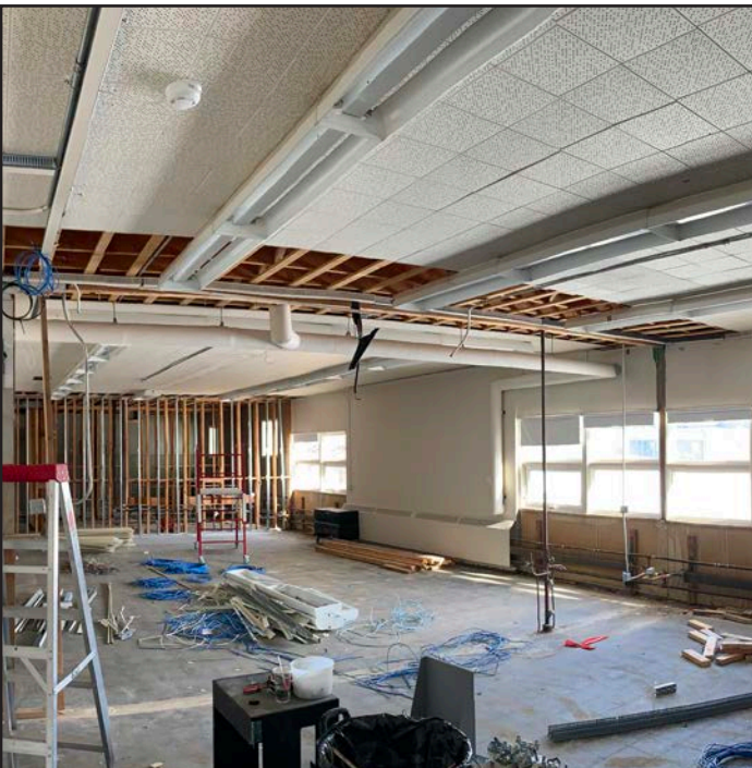
Town of Westlock Heritage Building Renovations Interworks Contracting Ltd.
